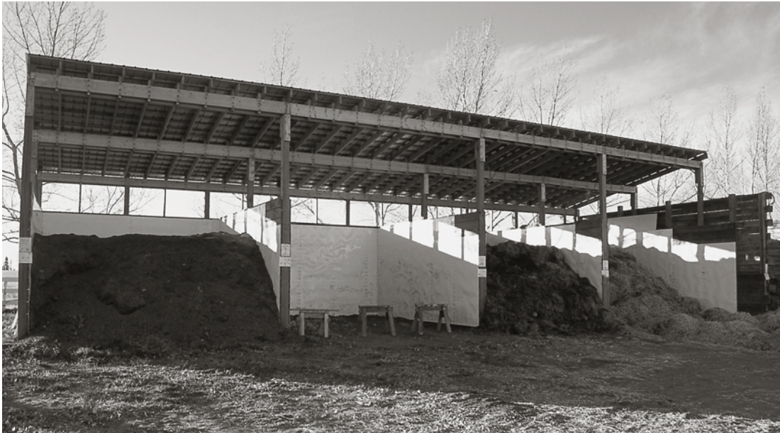
Figure 14. Multiple bin composting system.
