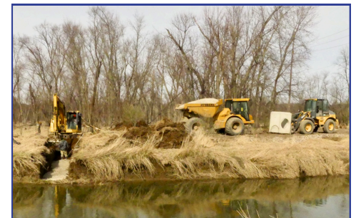
Construction in progress at Killbuck Creek
